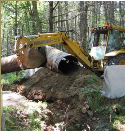
Allan Tufts and Aaron Theriau removing the old culvert at Square Camp Brook
